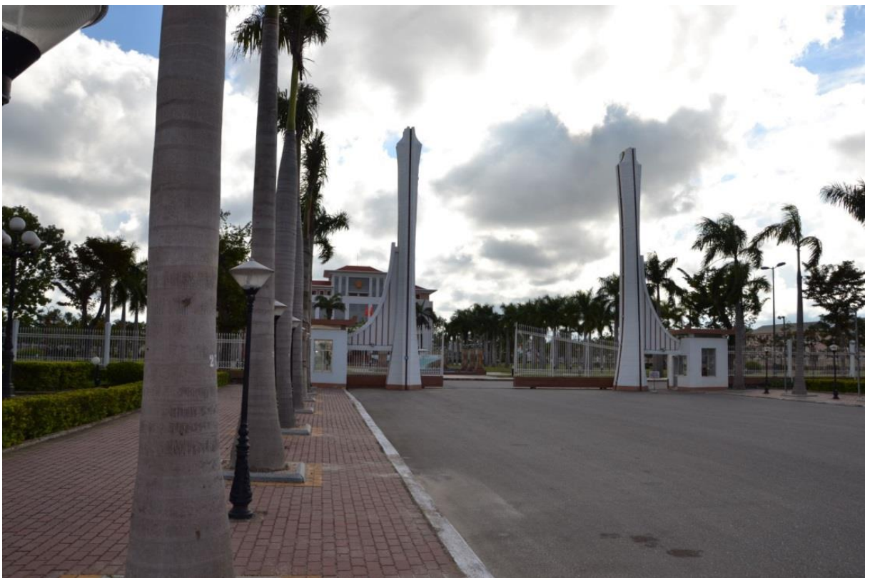
Figure 9 Administrative architecture: Main building of People's Committee in Tam Kỳ
